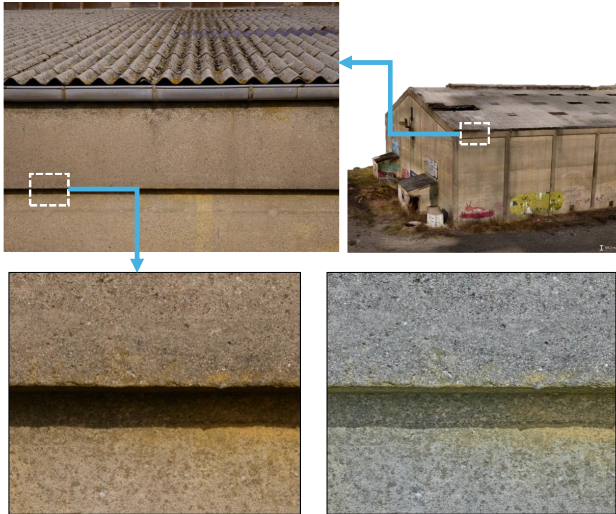
Figure 4: To extract features in the multi surface objects, some parts of the object could be hidden in the shadow areas (left) and where high dynamic range helps an advanced radiometric adjustment (right) to balance these areas
