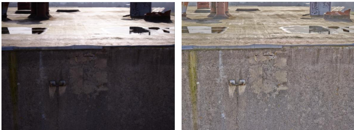
Figure 6: Raw IIQ images of a roof and a façade of a building in a challenging illumination condition with high contrast between extremely bright and dark areas (left, raw image), and radiometrically adjustment via HDR capabilities (right, adjusted image)
