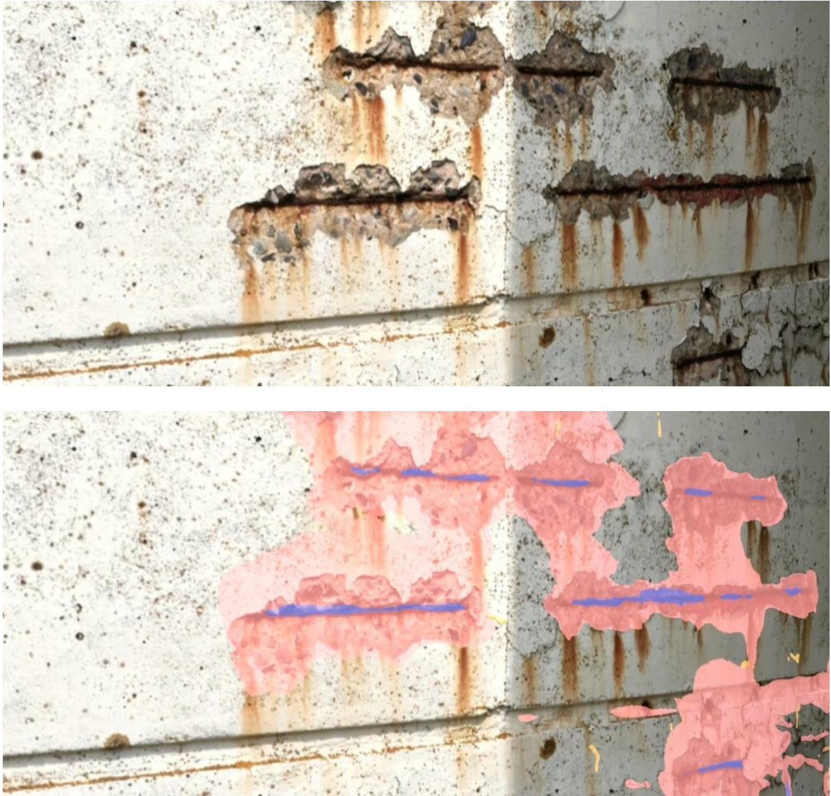
Figure 6: 3D mesh (up) and the results from crack detection (down), identifying classes of cracks (yellow), spallings (pink) and rust (purple), highlighting an emerging spalling
