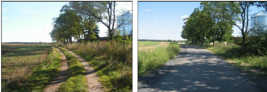
Fig 6. An example of post-merger management - reconstruction of an agricultural transport road. On the left, the state before land consolidation, on the right, the state after land consolidation. Source: [Ministry of Agriculture and Rural Development 2018].
