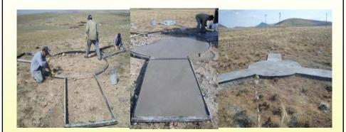
Photo: Poure concrete of GCP on the field.
