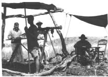
Fig.8 – Cartographic station, Boabá, 16 m (left); Plane table and alidad (up); Drawing the cartographic document (down)
