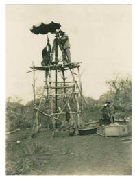
Fig.6b – projector; 10 m tower lined with straw; measuring angles (up, down, from left to right)
