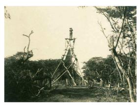
Fig.6 – Checking inter-visibilities from the top of a tree.
