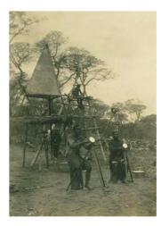
Fig.6a – part of the triangulation chain, N Tungluane tower and projectors, Landins pointing heliotropes
