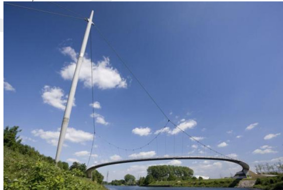
The award winning bridge at the Gelsenkirchen Grimberg port. (Foto: Malinowski)
