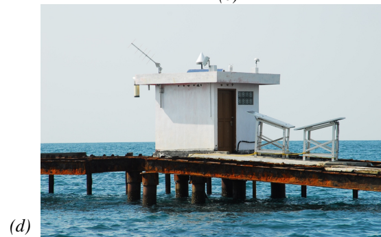
Figure 2. The IPGSN geodetic monument types: (a) on the top of concrete roof, (b) concrete pillar, (c) stainless-steel rod, and (d) on a tide gauge station. Photos are taken by Cecep Subarya.
