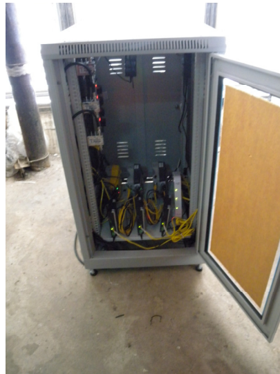
Figure 4: Installation of the GPS receivers and communication devices on the 65 th floor
