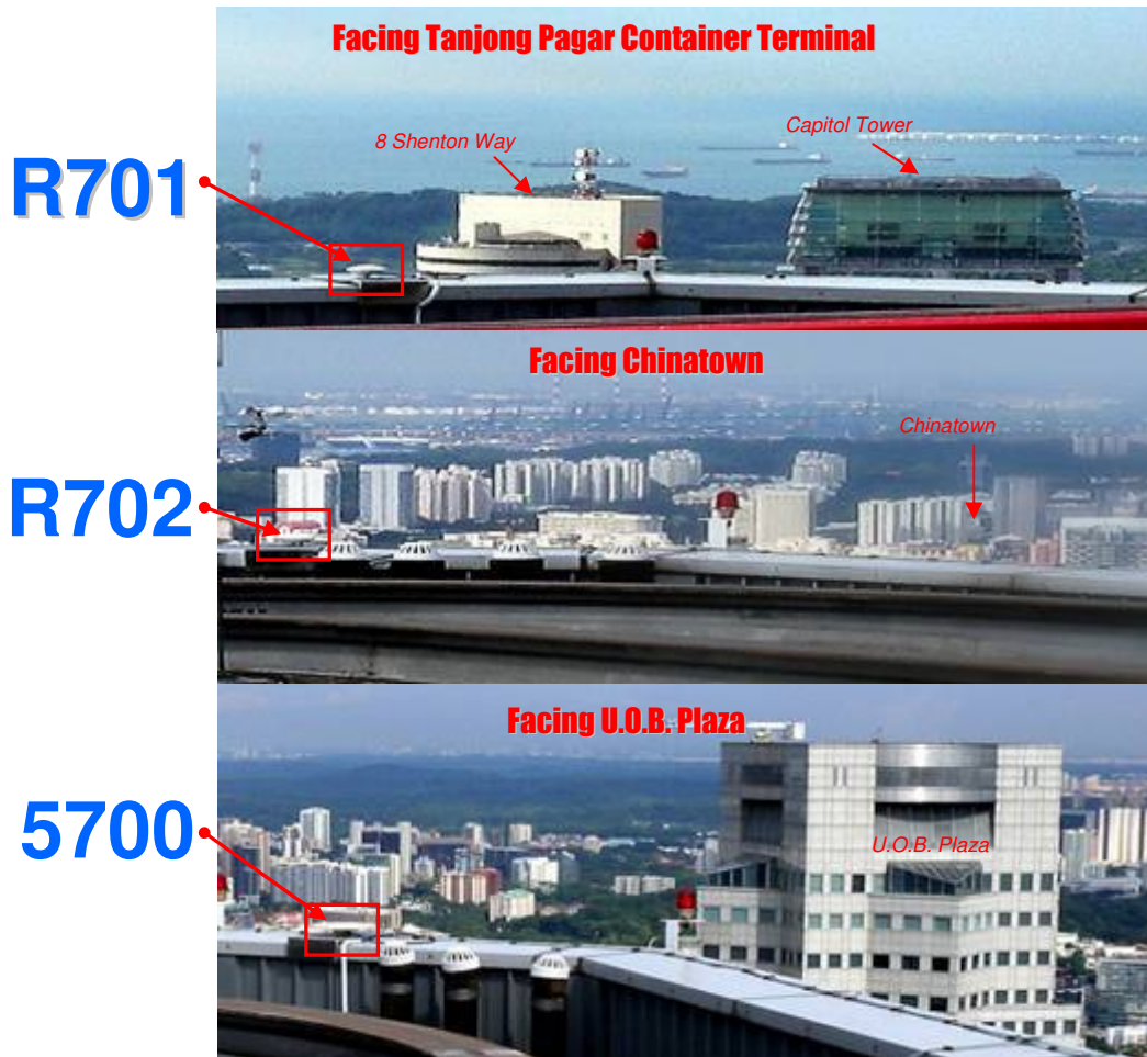
Figure 3: Installation of the 3 GPS antennas on the roof-top of Republic Plaza
