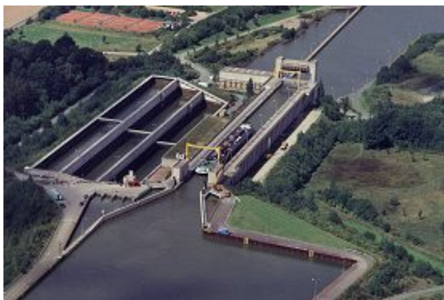
Fig. 1: Aerial view of lock Uelzen I
