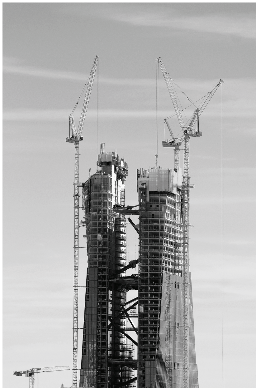
Figure 5 NEP Twin Towers, Frankfurt (Walter Wunderlich, 2011)
