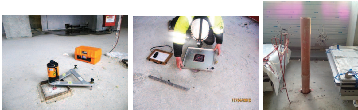
Figures 1 to 3 Laser plummet, transparent grid plate, pipe protection (Almesberger, 2014)
