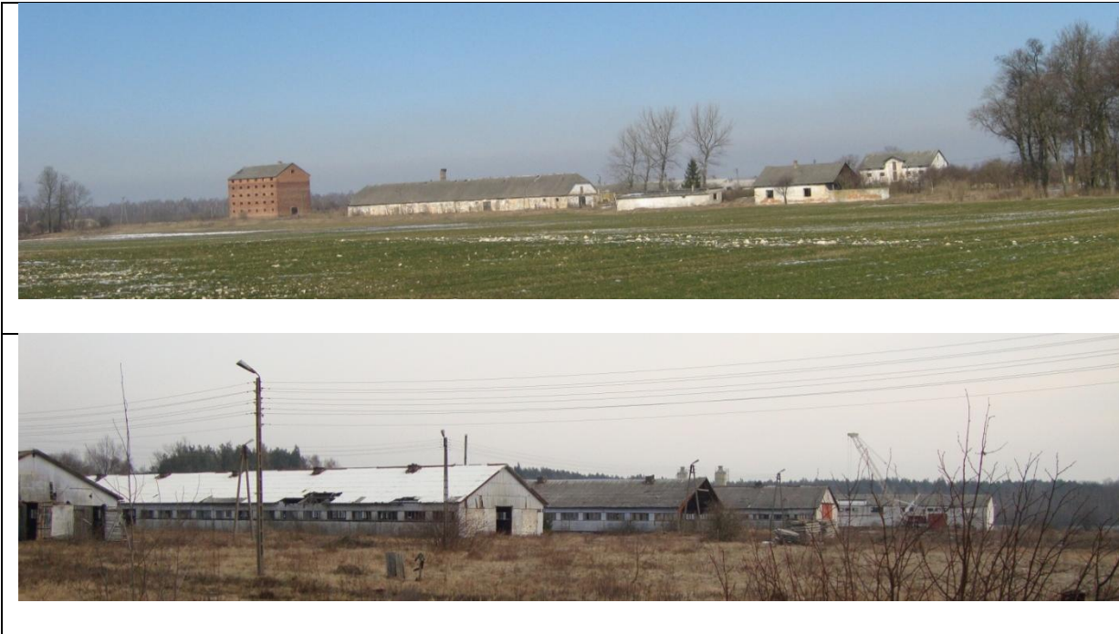
Farm buildings of ex-PGR farms
