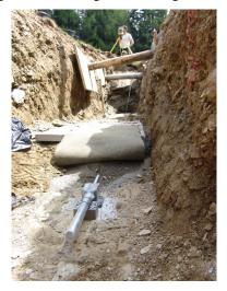
Figure 4 - Sensor S2 whilst embedding
