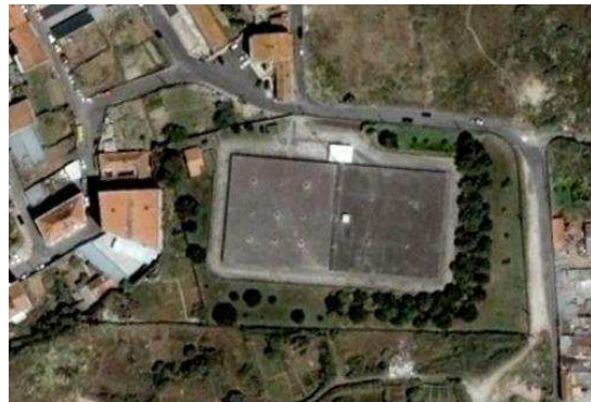
Figure 1 – Water tank in Alto Lumiar (Google Earth imagery)
