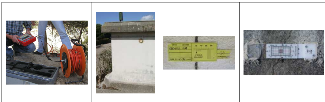
Figure 5 – Geotechnical instrumentation: inclinometers, tiltmeters, uniaxial and biaxial fissurometers.
