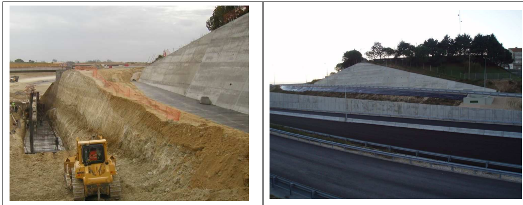
Figure 10 – Photo of the site during and after final works conclusions.
