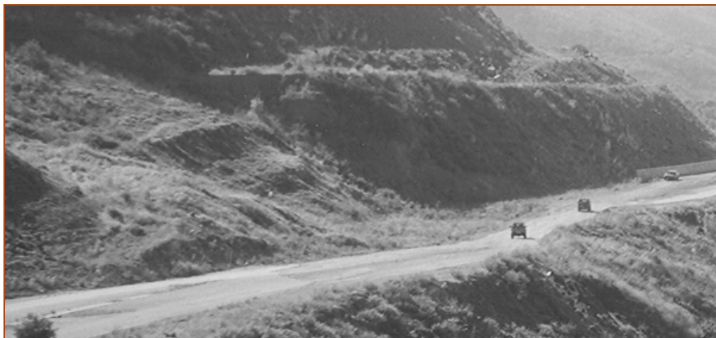
Photo 3: The cliff at the side of the national road
